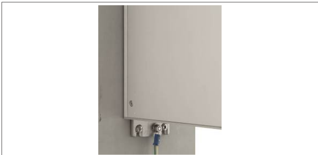
Figure 37: Connecting the ground cables
