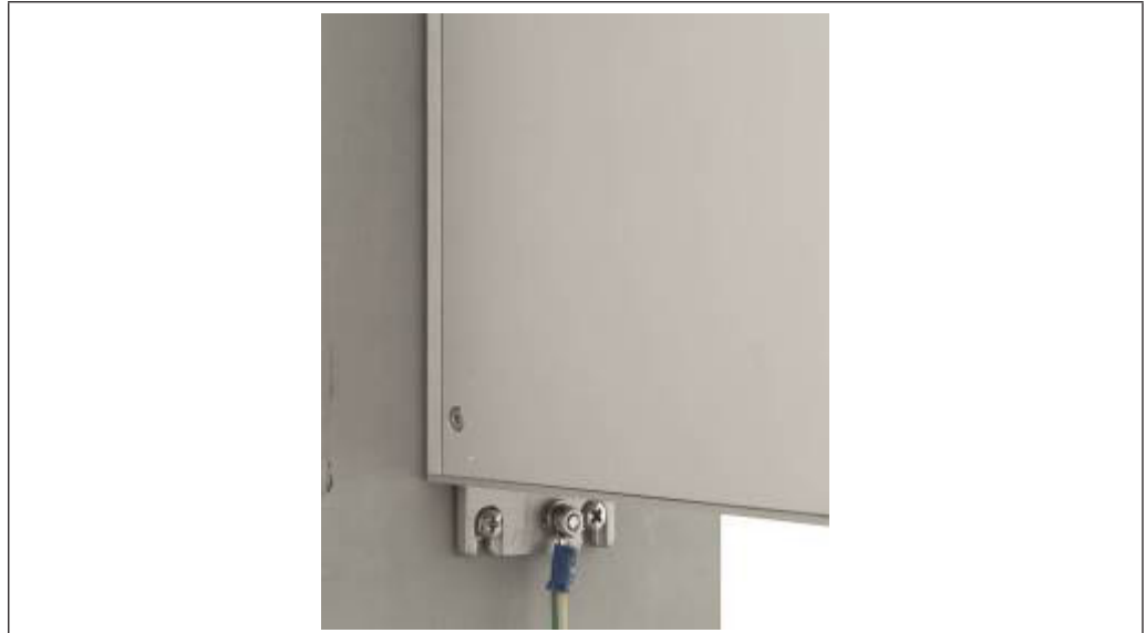
Figure 30: Grounding detail
